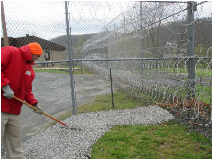
Correctional Industries at Denmar Correctional Center receives fence upgrades
