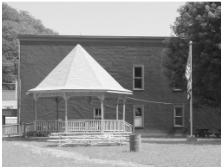
Gazebo constructed by DCC inmates for the Town of Marlinton.
