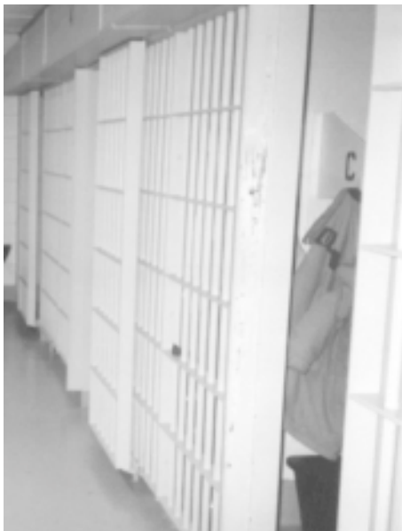
The typical Cell Block at OCCC.
