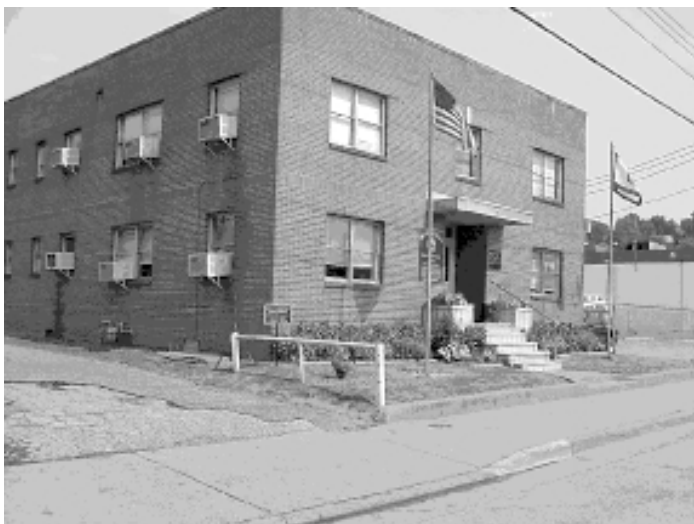
Front view of CWRC.
