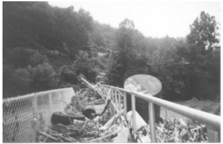
An example of flood damage cleaned up by BCC inmates in Southern WV.
