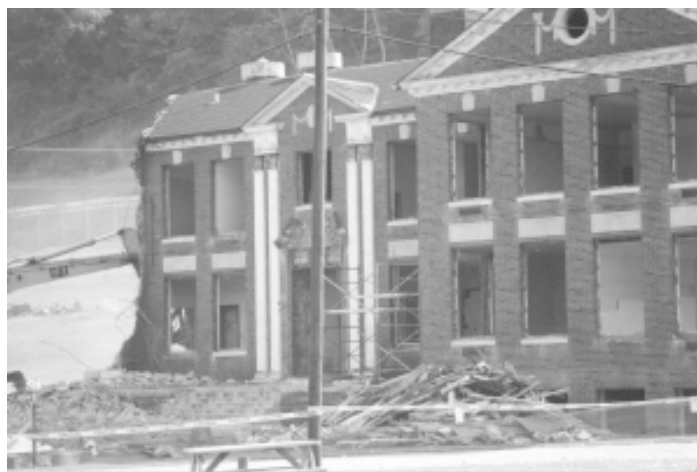
Examples of the ongoing construction and renovation at SMCC.
