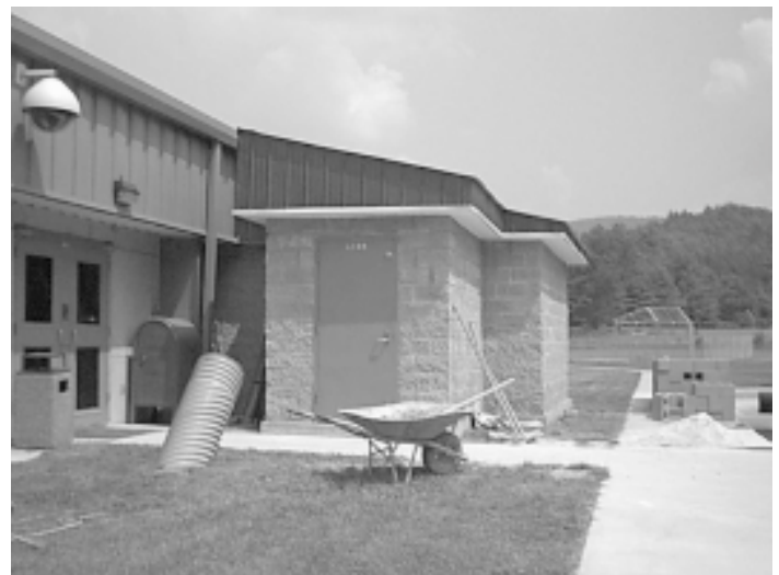
New Armory under construction at ACC.
