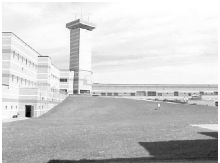
Rear View of the MOCC Administration Building
