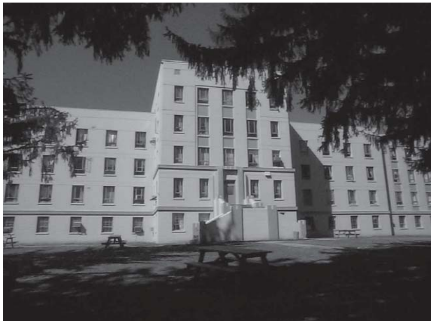
Denmar Correctional Center
