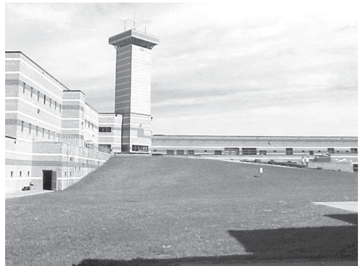
Rear View of the MOCC Administration Building
