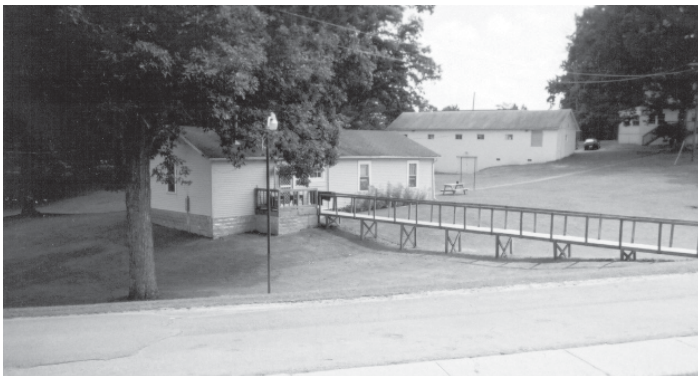
BCC - Building 3 Male Housing Unit
