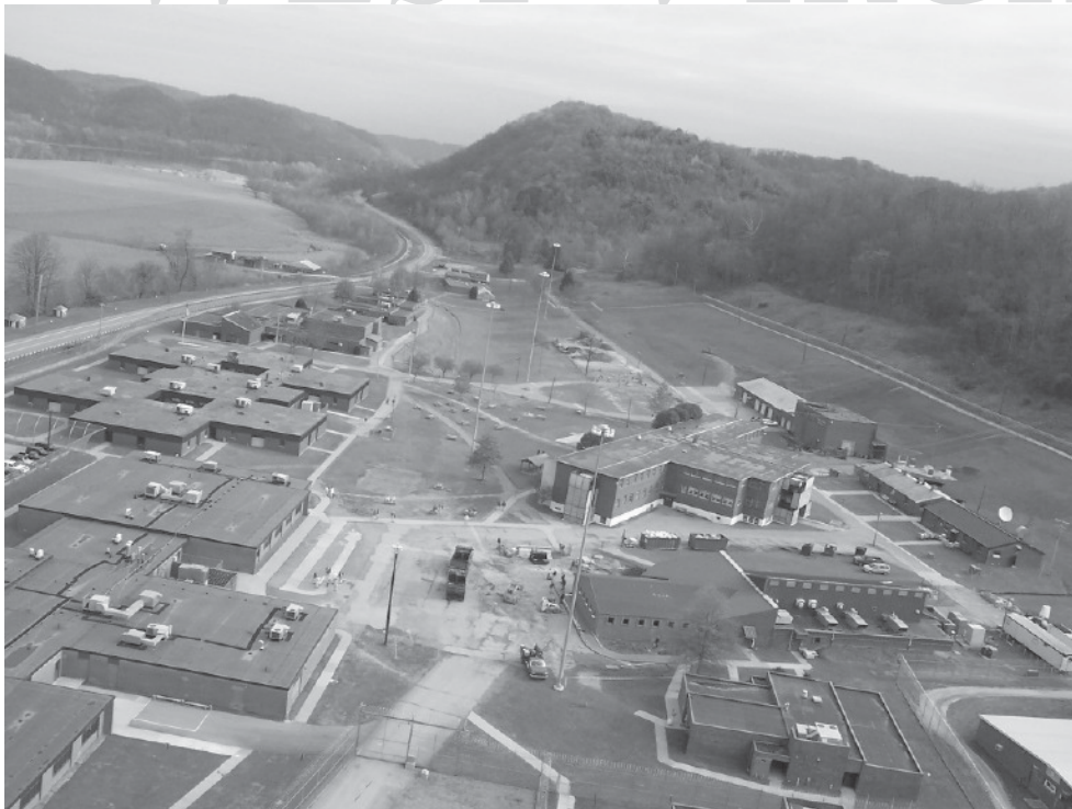
St. Marys Correctional Center St. Marys, WV
