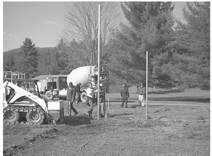
Construction on ACC Security Fence Begins
