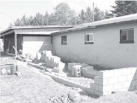
Construction on New HCC K-9 Kennel
