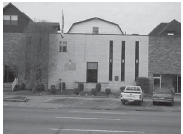
Huntington Work Release Center
