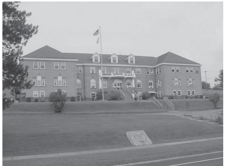
Pruntytown Correctional Center
