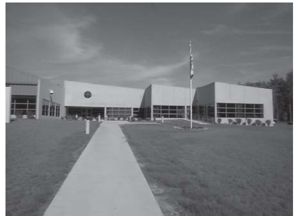
Anthony Correctional Center
