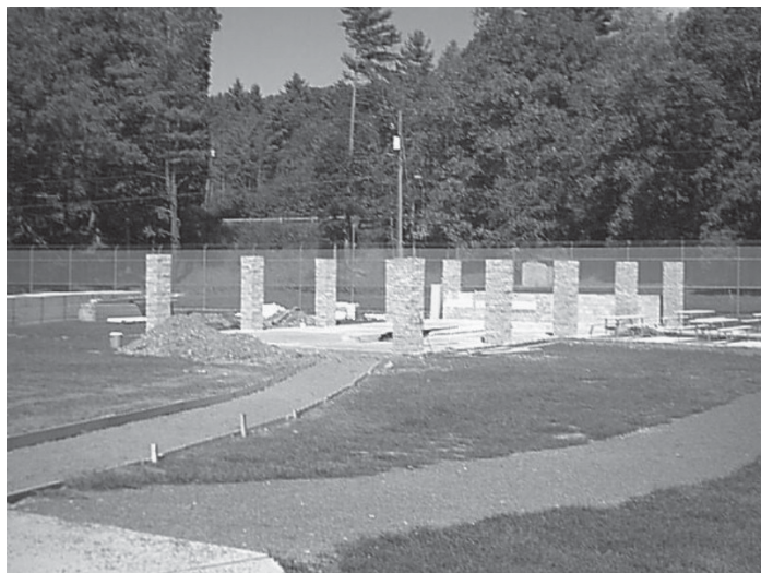
ACC Picnic Shelter and Walking Track under construction
