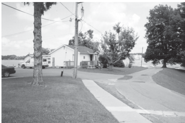
BCC-Building 2 Male Housing Unit
