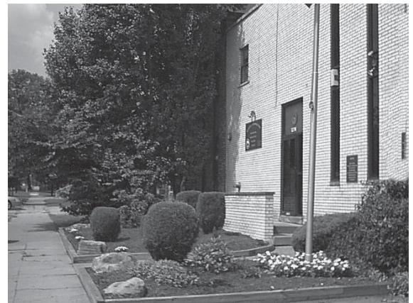
Huntington Work Release Center
