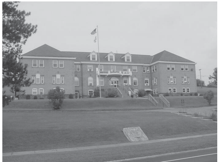
Pruntytown Correctional Center
