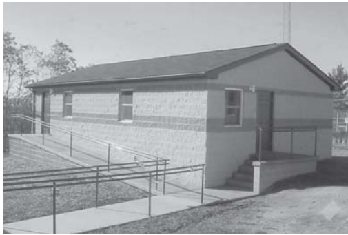
Multi Purpose Building built by Construction Class
