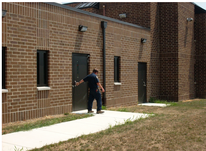
MCC's New Addition
